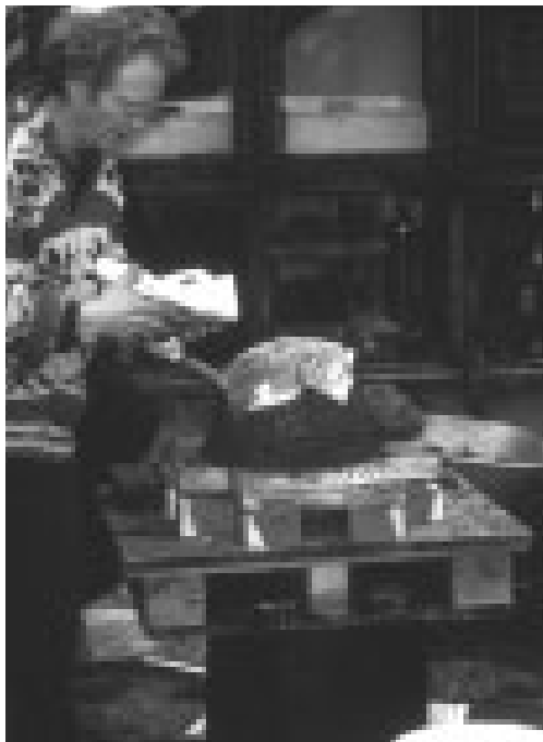
3 stages in building an earth-oven. 1. Put newspaper on the sand form. 2. Put earth on the form. 3. Cut out the door.
