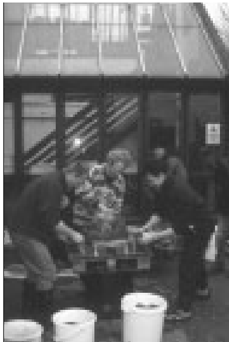
3 stages in building an earth-oven. 1. Put newspaper on the sand form. 2. Put earth on the form. 3. Cut out the door.
