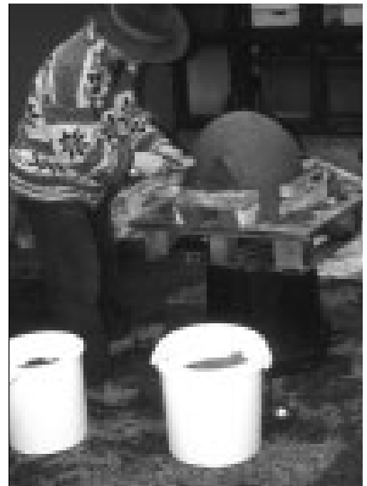
3 stages in building an earth-oven. 1. Put newspaper on the sand form. 2. Put earth on the form. 3. Cut out the door.
